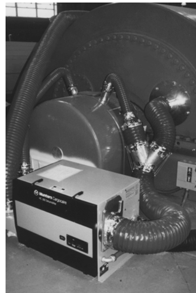
Figure 12. A Munters rental dehumidifier setup to protect the hotwell of the condenser in a power generation plant. Dry air circulates through the equipment, preventing corrosion from occurring. Courtesy Munters Moisture Control Services.
