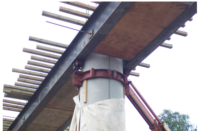
Photograph 5-393-200-1 — A view of friction collar used to support the falsework for the construction of a concrete pier cap.
