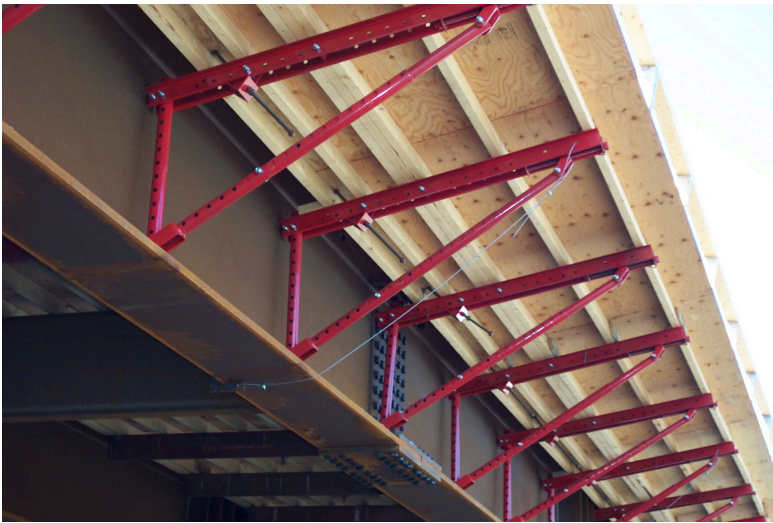
Photograph 5-393-200-3 — A close-up of over hang brackets used to support the concrete overhang. Shown used on a bridge with steel beams.
