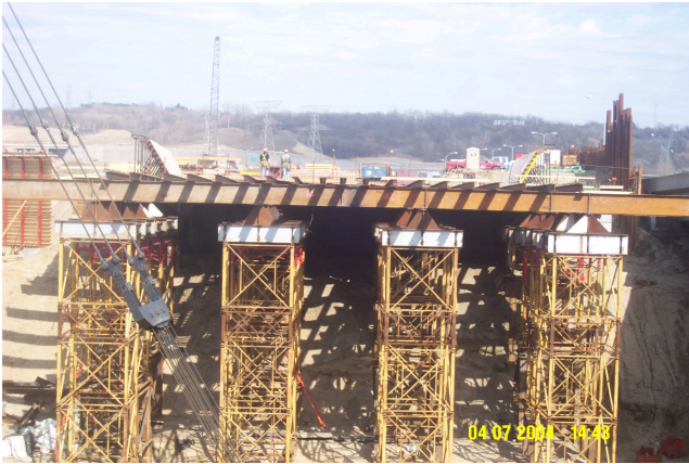
Photograph 5-393-200-4 — A view of the use of tubular steel scaffolding used as falsework for the construction of a concrete slab-span bridge.
