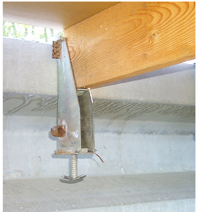
Photograph 5-393-200-2 — A close-up of a typical steel joist hanger used as a bracket to support the ends on joists used for falsework for the interior bays roadway slab construction.
