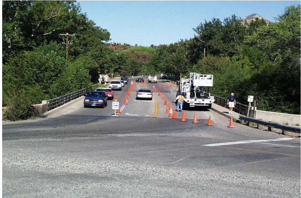
Figure 2.3.1 Temporary Traffic Control Operation
