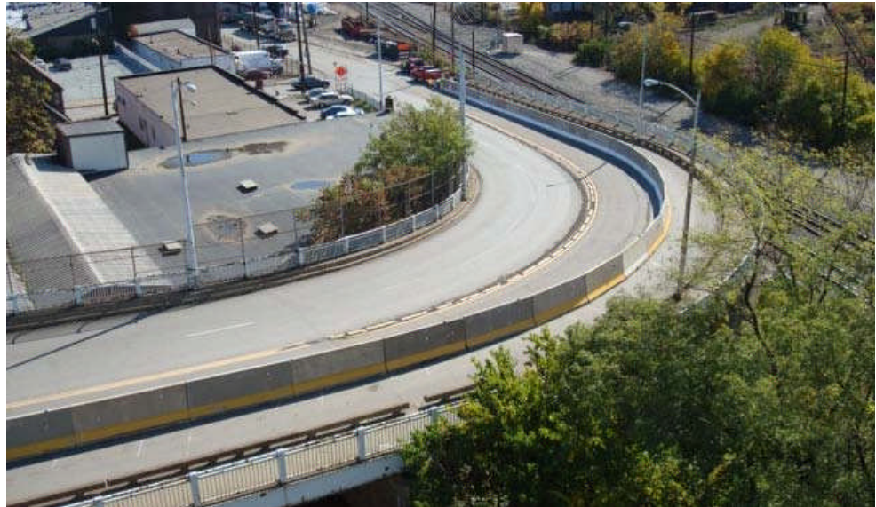
Figure 2.3.13 Temporary Traffic Barriers
