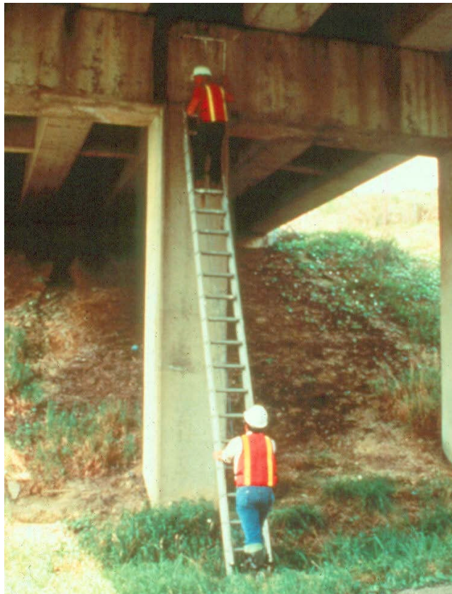
Figure 2.2.8 Proper Use of Ladder
