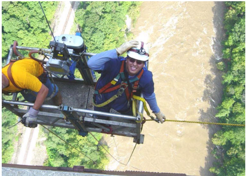
Figure 2.2.6 Inspector with Safety Harness with a Lanyard
