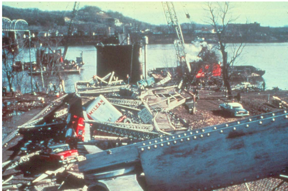
Figure 1.1.2 Collapse of the Silver Bridge
