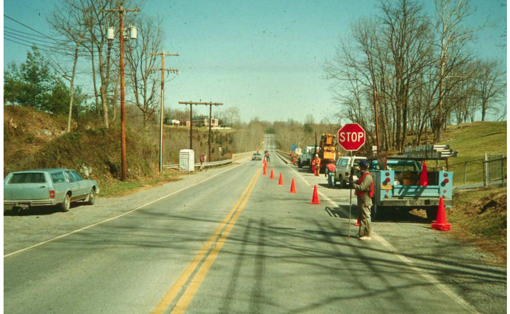
Figure 2.1.4 Temporary Traffic Control Operation
