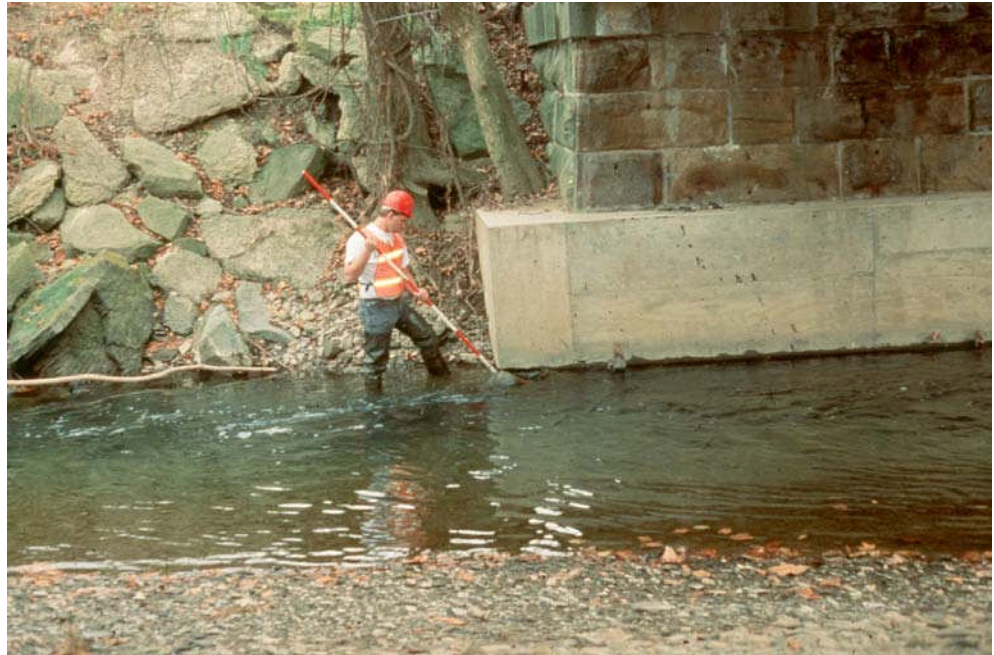
Figure 2.1.5 Inspection for Scour and Undermining
