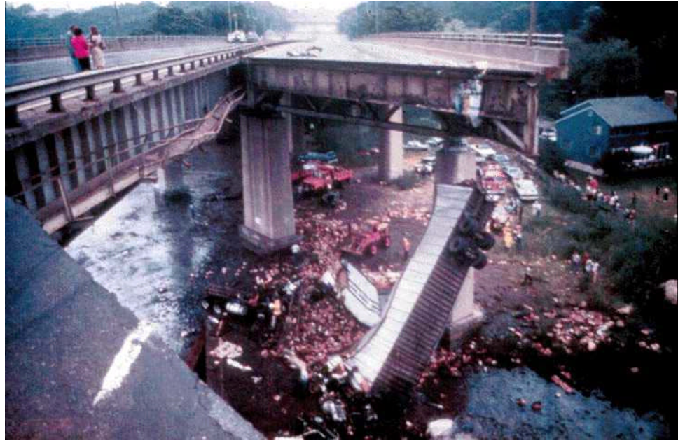
Figure 1.2.1 Mianus Bridge Failure
