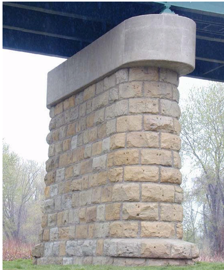
Figure 3.1.76 Solid Shaft Pier
