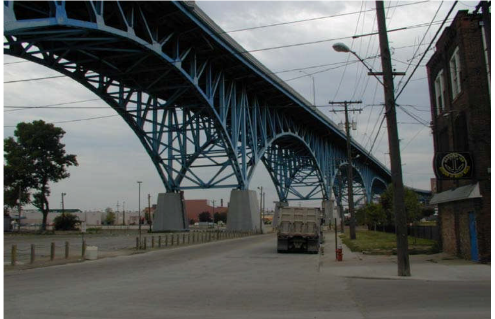
Figure 3.1.52 Deck Truss Bridge
