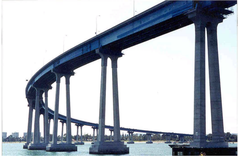
Figure 3.1.48 Curved Girder Bridge
