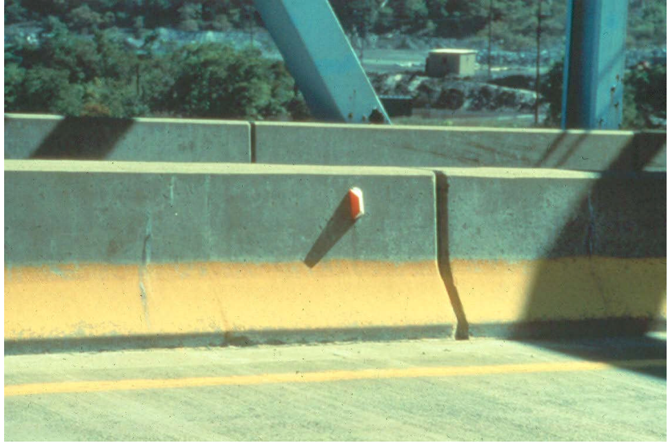
Figure 3.1.40 New Jersey Barrier
