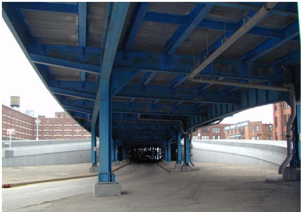
Figure 3.1.80 Column Bent
