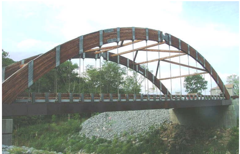
Figure 3.1.55 Through Arch Bridge
