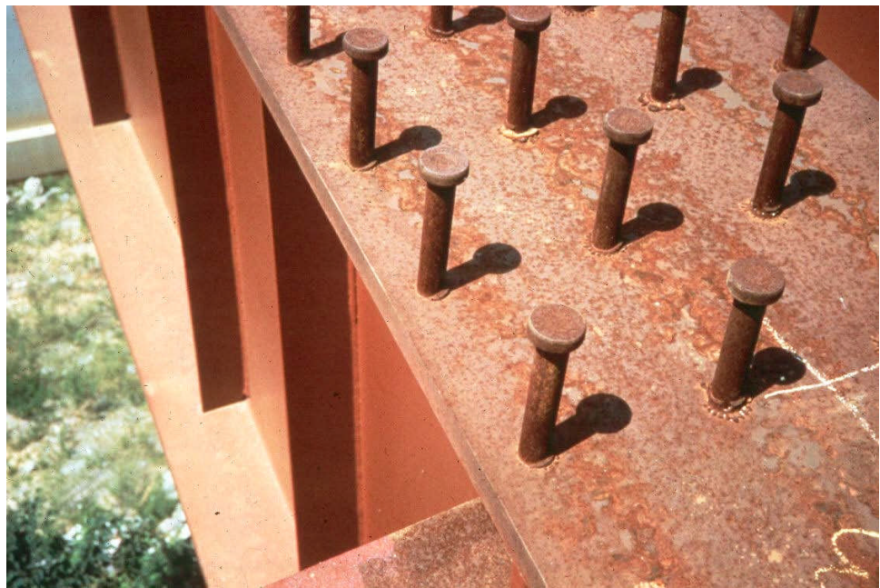
Figure 3.1.31 Shear Studs on Top Flange of Girder (before Concrete Deck is Placed)
