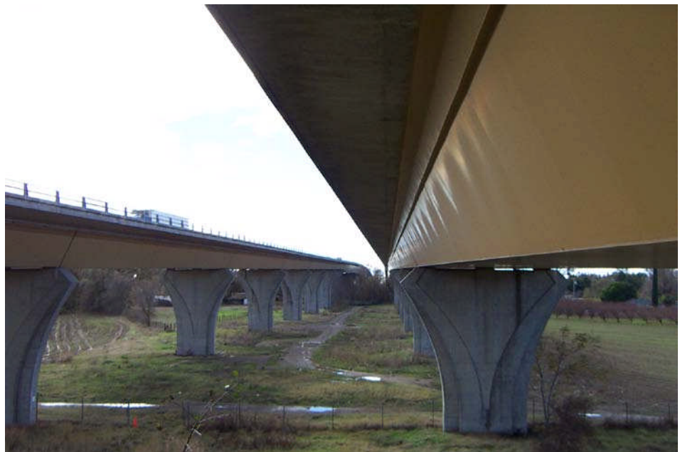
Figure 3.1.51 Box Girder Bridge
