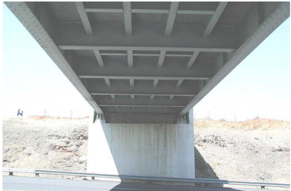
Figure 3.1.47 Girder Floorbeam Stringer Bridge
