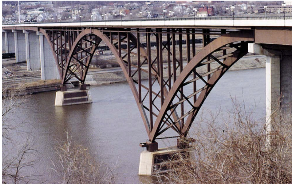
Figure 3.1.64 Main Supporting Members of Deck Arch
