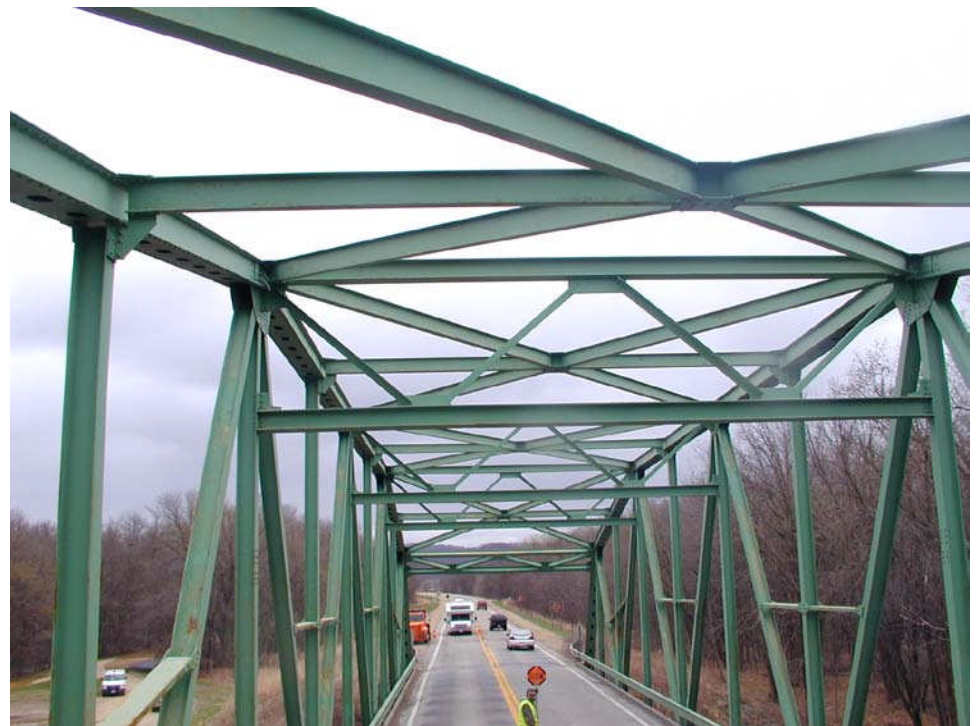
Figure 3.1.67 Top Lateral Bracing and Sway Bracing
