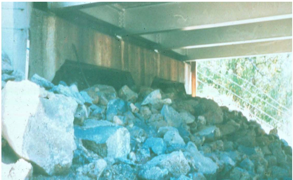
Figure 3.1.73 Spill-Through or Open Abutment
