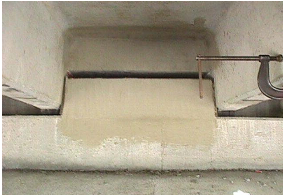
Figure 3.1.49 Tee Beam Bridge
