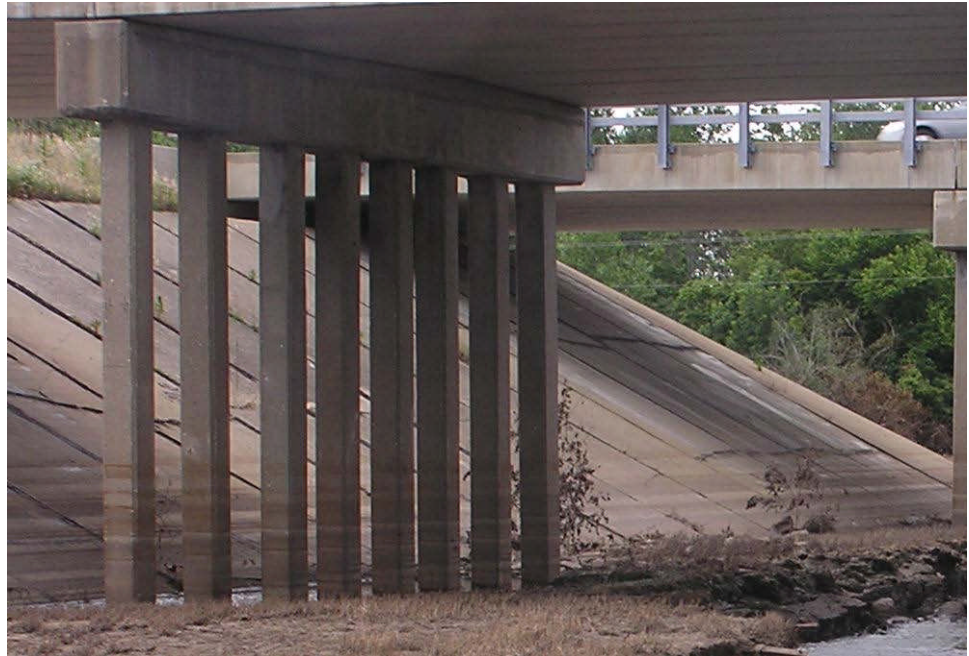
Figure 3.1.10 Concrete Pile Bent
