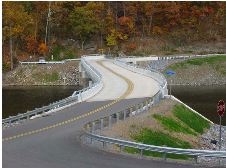
Figure 3.1.28 Bridge Deck with a Smooth Riding Surface
