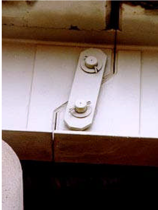
Figure 3.1.26 Pin and Hanger Assembly
