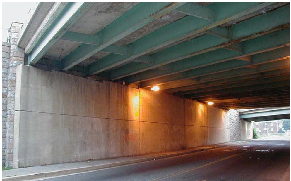
Figure 3.1.71 Cantilever Abutment (or Full Height Abutment)
