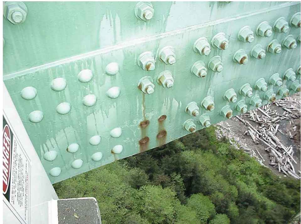
Figure 3.1.24 Shop Rivets and Field Bolts
