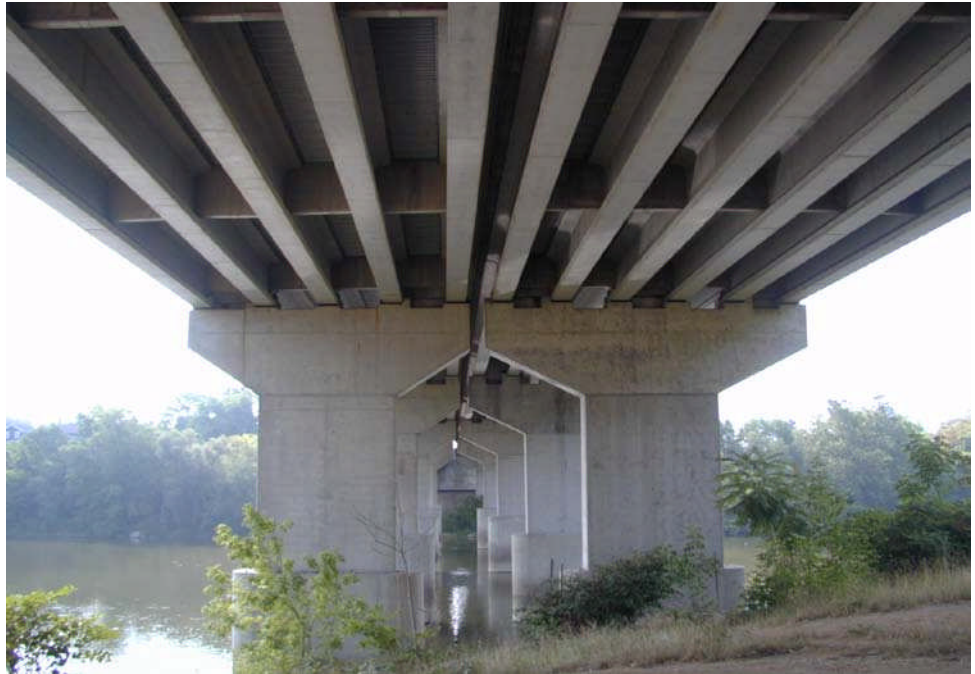
Figure 3.1.79 Cantilever or Hammerhead Pier
