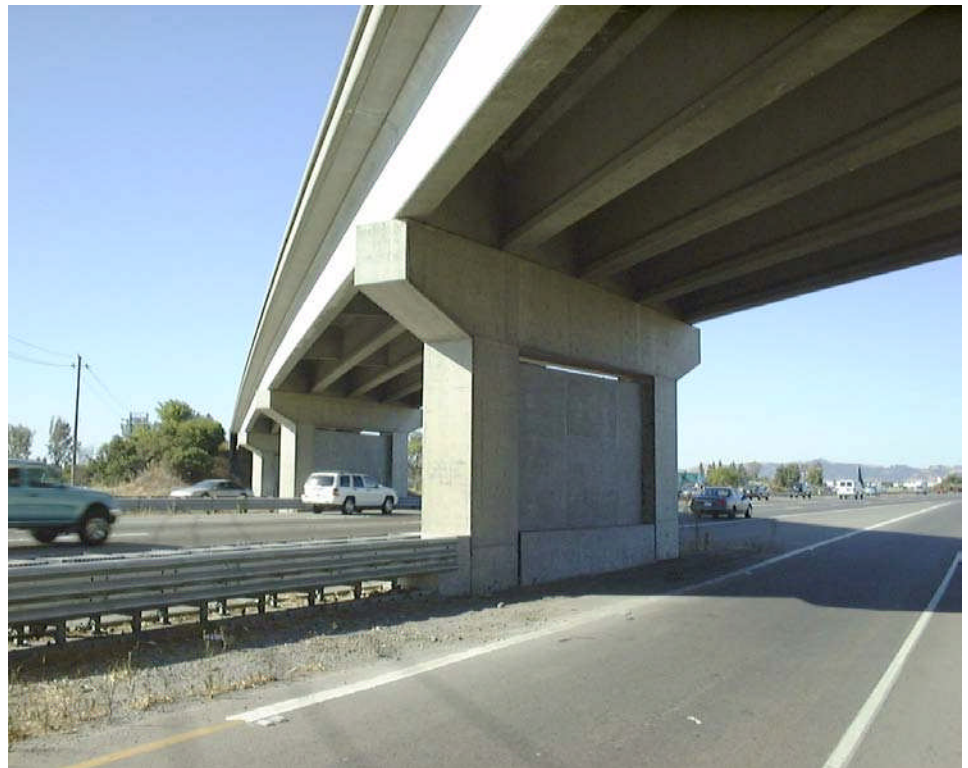
Figure 3.1.78 Column Pier with Web Wall and Cantilevered Pier Caps
