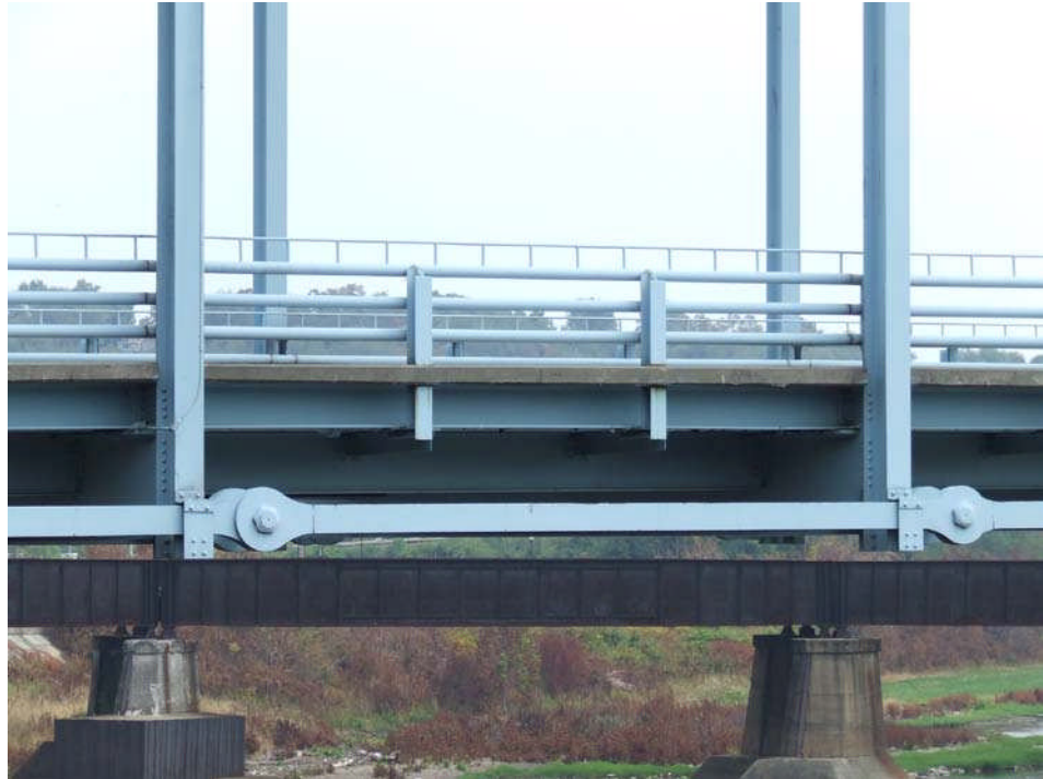
Figure 3.1.22 Pin-Connected Eyebars
