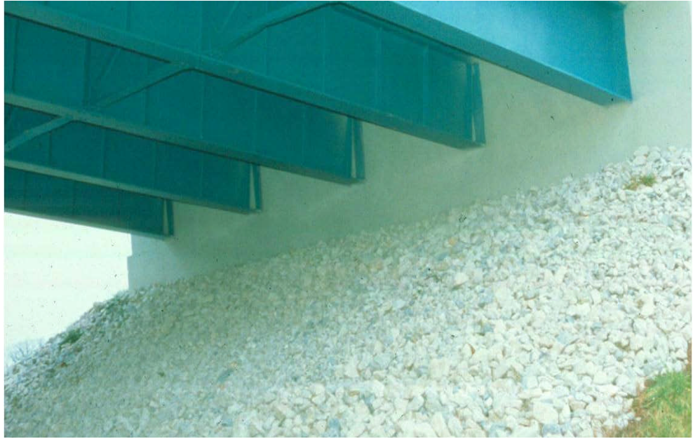
Figure 3.1.74 Integral Abutment
