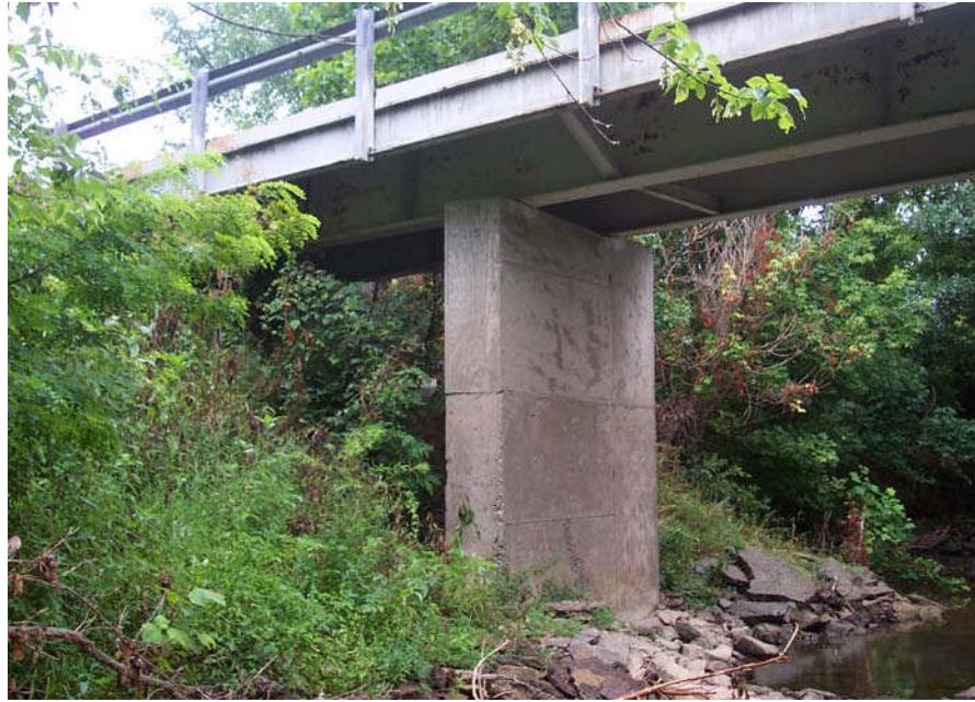
Figure 3.1.75 Solid Shaft Pier
