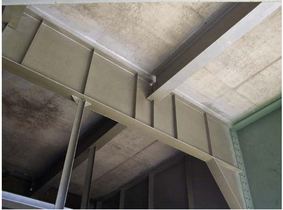
Figure 3.1.29 Underside View of a Bridge Deck
