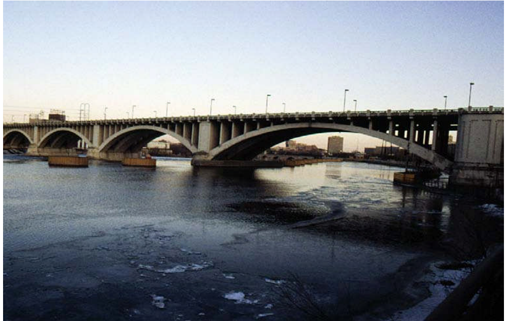
Figure 3.1.54 Deck Arch Bridge
