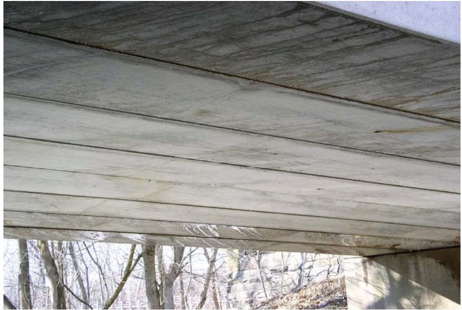
Figure 3.1.50 Adjacent Box Beam Bridge
