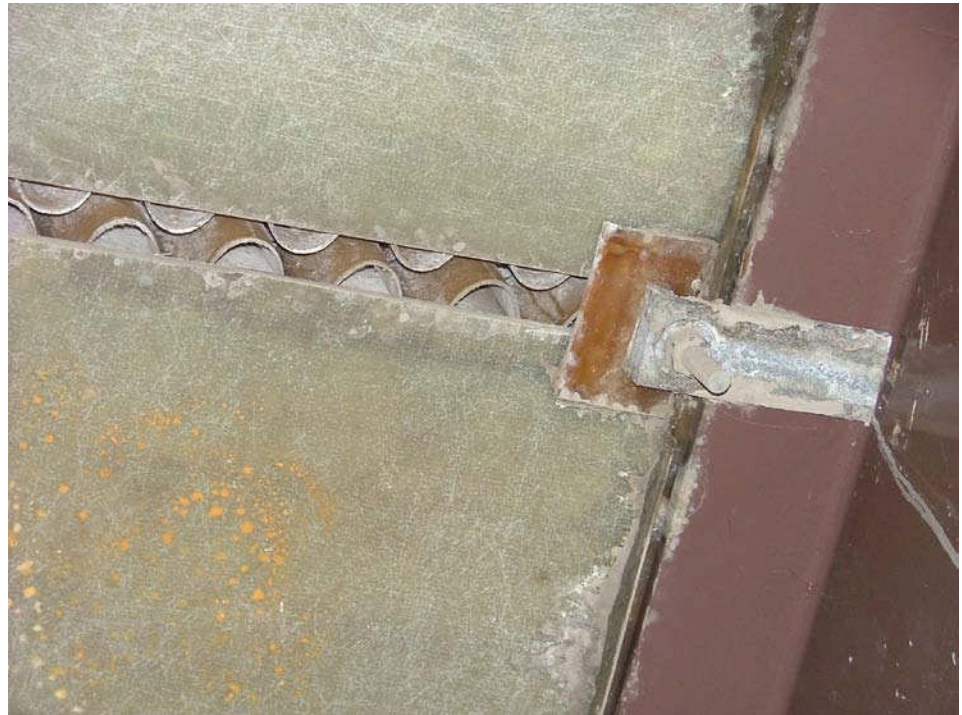
Figure 3.1.35 Fiber Reinforced Polymer (FRP) Deck
