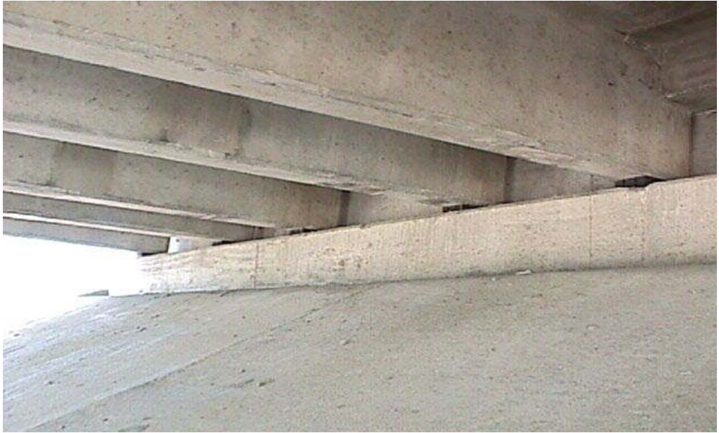
Figure 3.1.72 Stub Abutment
