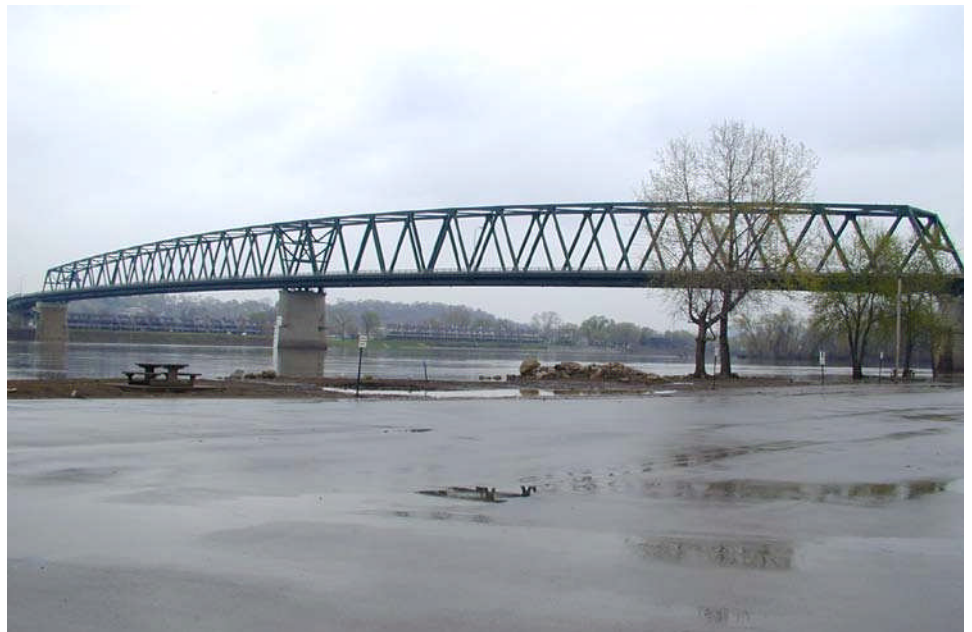
Figure 3.1.53 Through Truss Bridge
