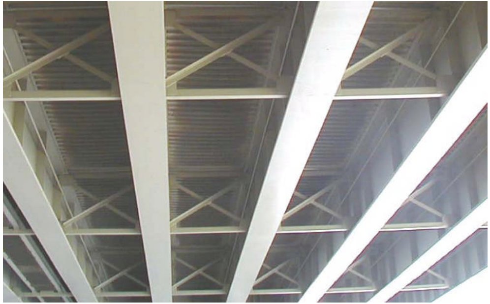
Figure 3.1.66 Cross or X-Bracing
