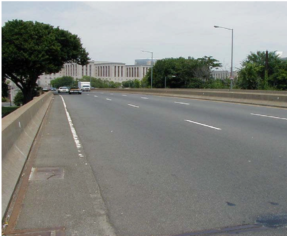
Figure 3.1.36 Asphalt Wearing Surface on a Concrete Deck
