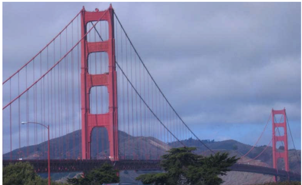
Figure 3.1.19 Cable-Supported Bridge: Suspension Cables and Hangers
