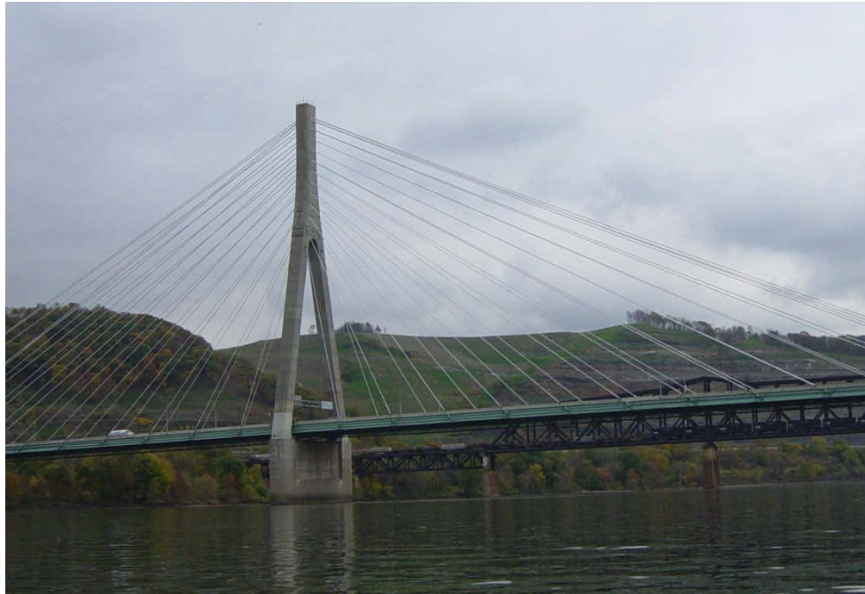
Figure 3.1.20 Cable-Supported Bridge: Cable Stayed
