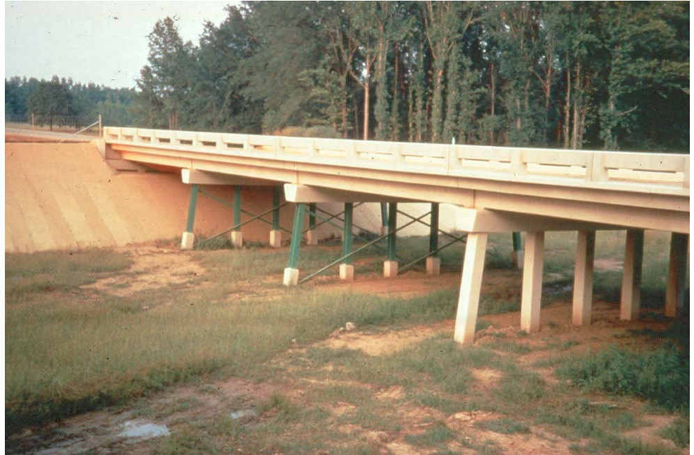
Figure 3.1.81 Pile Bent
