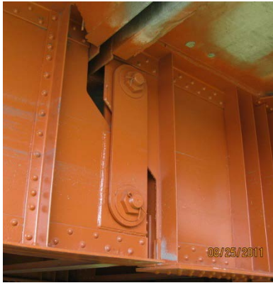
Pin and Hanger Assembly on a Riveted Steel Girder Bridge
