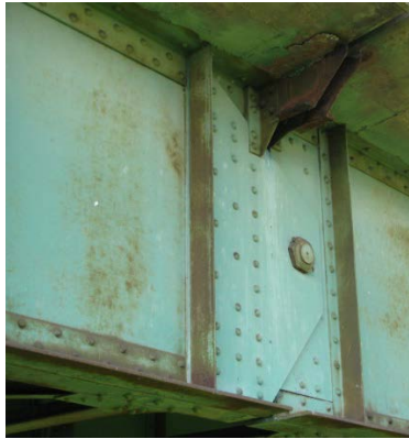
Fixed Pin Assembly on a Riveted Steel Girder Bridge
