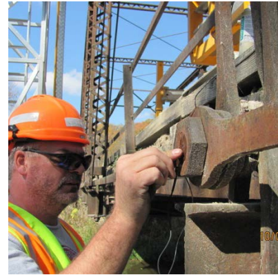
Ultrasonic Examination of a Pinned Truss Connection
