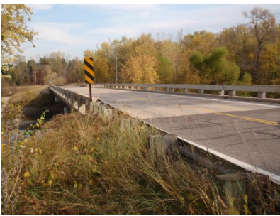
1. Roadway across Bridge
