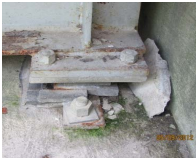
Sliding plate bearing near the design limits of expansion
