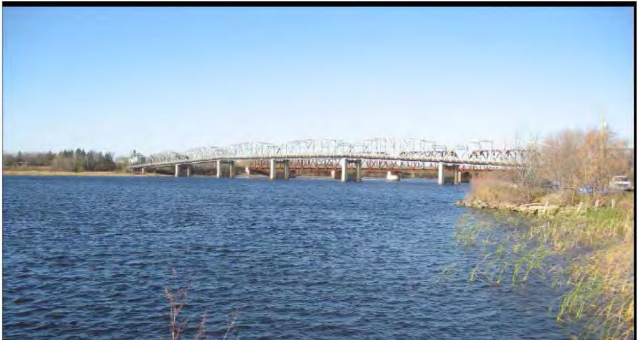
Figure 1: View of Bridge 9412 from the east
