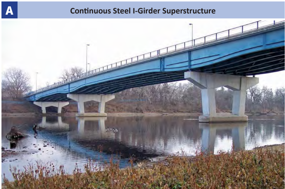
Camden Bridge, Minneapolis, MN
