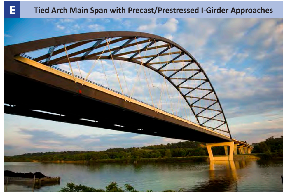
Blennerhassett Bridge, Belpre, OH & Parkersburg, WV
