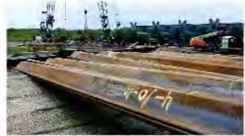
Figure 3. Drying will also kill aquatic organisms. Lay out materials to dry in the proper time. Drying times vary by species. Inspect after drying period is over. Photo credit: Dwayne Stenlund, MnDOT
