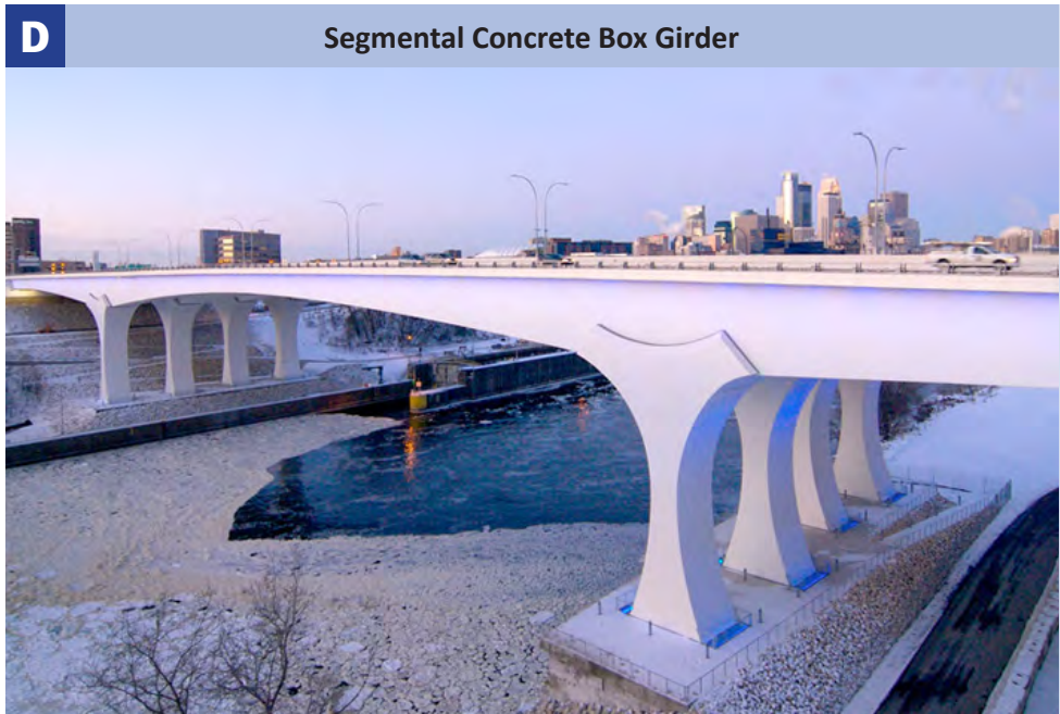
I-35W Saint Anthony Falls Bridge, Minneapolis, MN
