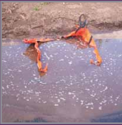
Flooded inlet protection.
