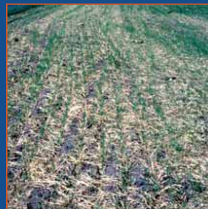
Temporary seed mix installation with a properly applied mulch.
