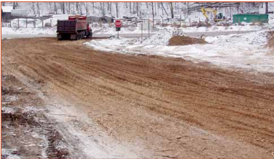
Woodchip stabilized tracking pad.
