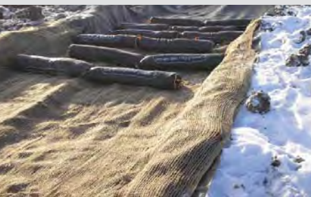
Flocculant treatment system with jute netting and erosion control log baffles
