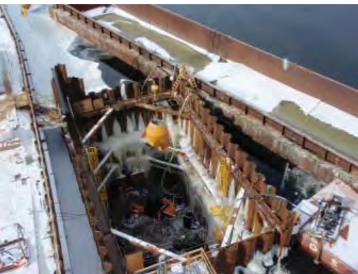
Ice buildup inside a cofferdam work area
