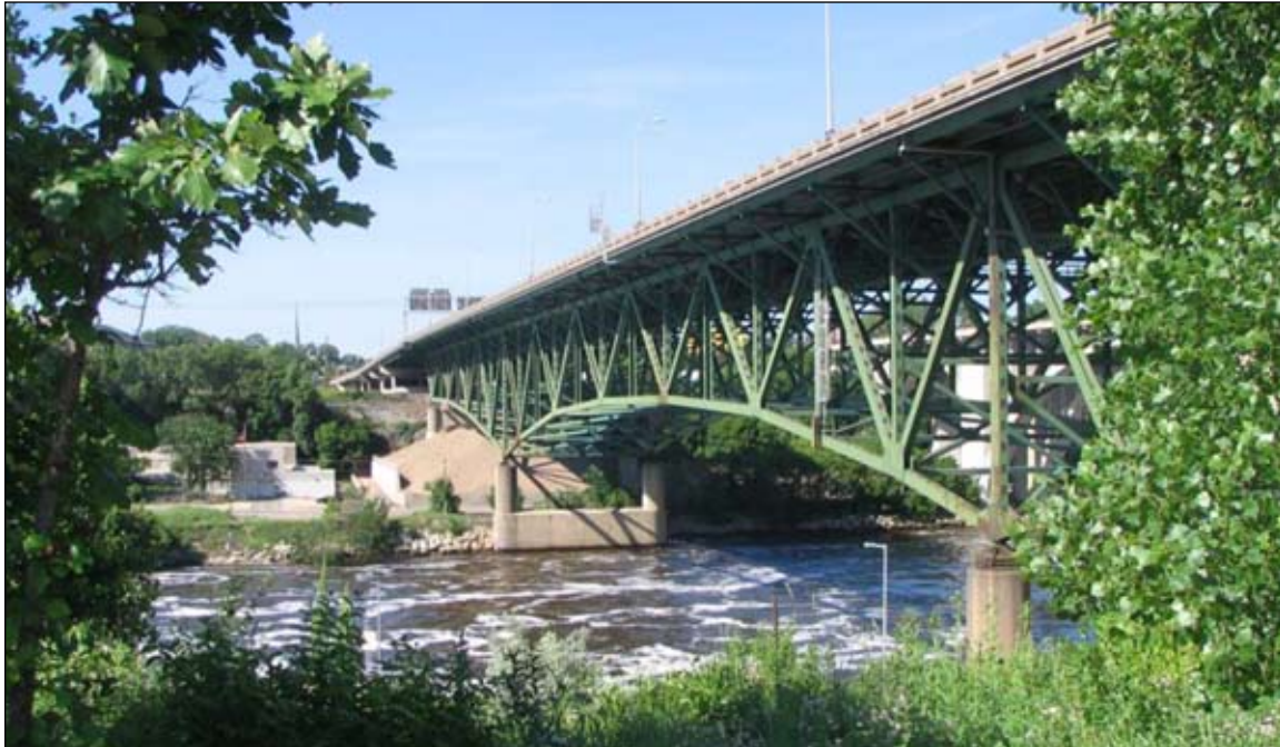
Figure 4. Center span of I-35W bridge, looking northeast. The center span is supported by pier 6 on the near (south) riverbank and pier 7 on the far (north) riverbank.
