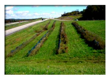
**Project Description:** Keeping snow and ice off of windswept areas of the roadway can be aided by the installation of a traditional snow fence, tree and shrub planting, and by leaving standing corn rows in farm fields. In roadway ditch rights of way where these methods are not an option or have proved to be too expensive to implement, the district will plant a 10-foot-wide swath of tall native gasses and a 5-foot-wide strip of a perennial cone wildflower mix to serve as a windbreak.
