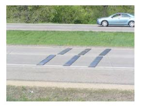
**Project Description:** RoadQuake temporary, portable rumble strips alert drivers to reduce speed. This device can be used in highway and road construction applications, including short-term work zones, temporary lane closures or law enforcement checkpoints. RoadQuake is a temporary device and does not require adhesives or fasteners for installation.
