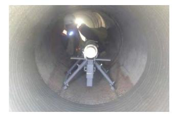
**Project Description:** Thousands of centerline roadway pipes in District 6 are deteriorating due to large-scale rust, holes and pipe separation. There is an increased risk of culvert/roadway failures if these defects are not corrected, but it is cost-prohibitive to fully replace the pipes. A new culvert lining called the Centri-Pipe, a centrifugally cast concrete pipe, appears to be a cost-effective way to extend pipe life by 50 to 100 years.
