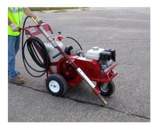
**Project Description:** Filling roadway cracks with crumb rubber or epoxy requires that the crack be blown clean and dry and heated before filling. This operation now requires a three-person crew with multiple pieces of equipment. To streamline this operation, the district will test the Crack Jet II, a self-contained heat lance, designed for an operator to walk behind, that uses hot air to dry moisture and blow cracks clean.
