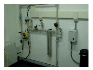
**Project Description:** The district will add a state-of-the-art material dispensing unit to its AccuBrine salt brine generators. The unit consists of a series of pumps equipped with flow meters that allow for accurate blending and dispensing of up to five different chemicals into either the tank on a plow truck or into larger tankers for distribution to other sites. A computer monitors and controls the mixture rate at which the pumps are flowing to give the operator an accurate mixture.
