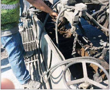
A sample of material is taken from microsurfacing machine for analysis by MnDOT lab.
