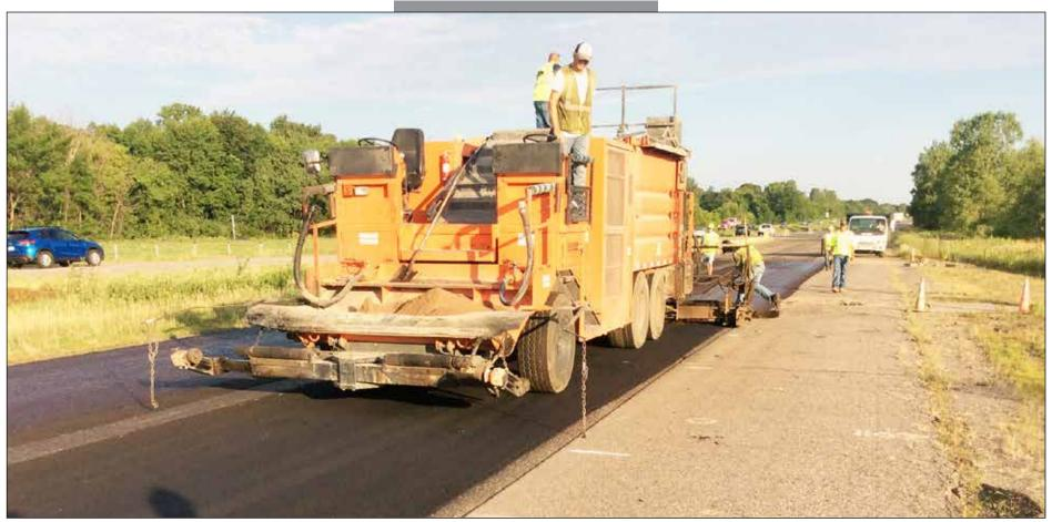
A section of MnDOT's MnROAD test track is microsurfaced as new National Road Research Alliance addresses troublesome paving issues to help DOTs nationwide.
